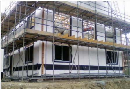
Bespoke preformed insulated DPC surrounds for openings supplied for use on German system building developments
